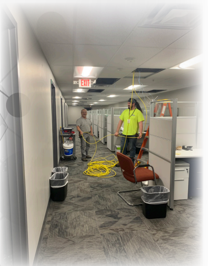
Fiber installation in Springfield
