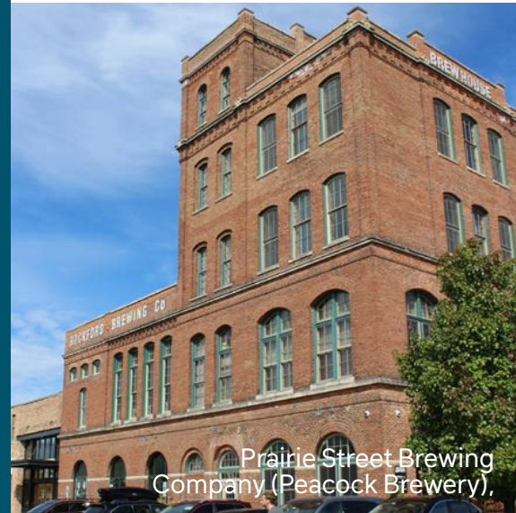
Embassy Suites (Ziock Building)
