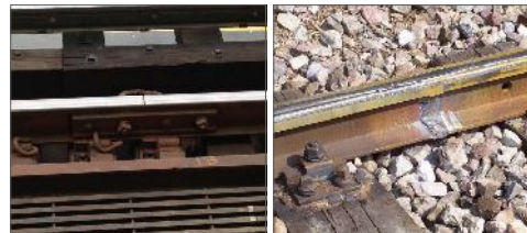
Jointed Rail versus Welded Rail
