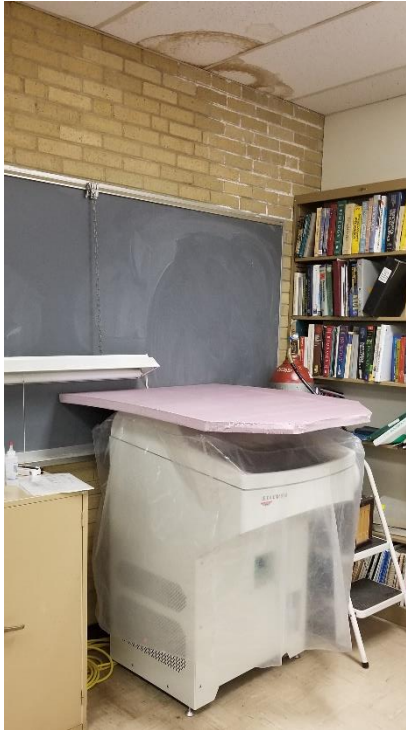
Water leak above cryostat (laboratory equipment)
