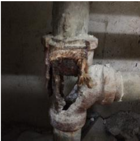
Pipe corrosion
