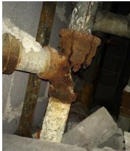
Pipe corrosion
