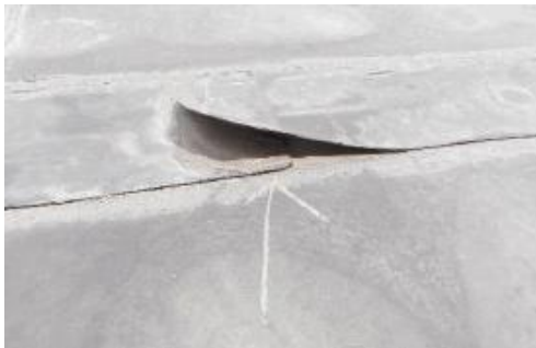
Seam delamination
