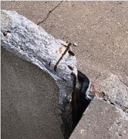
Concrete erosion
