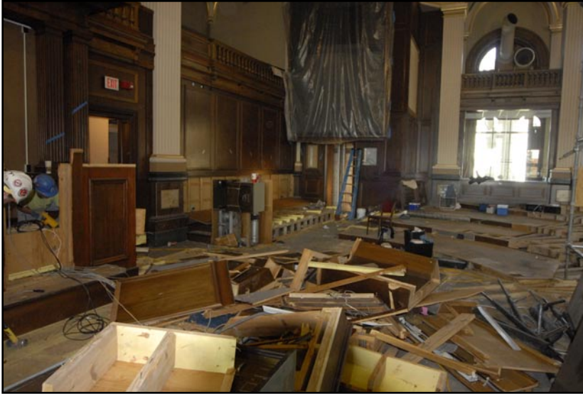
The chamber in the midst of demolition.
