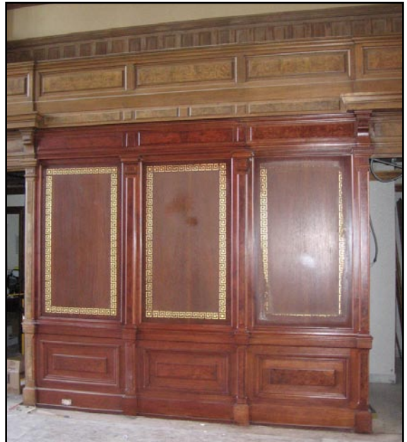
Newly refinished wood and existing wood on south wall of chamber.
