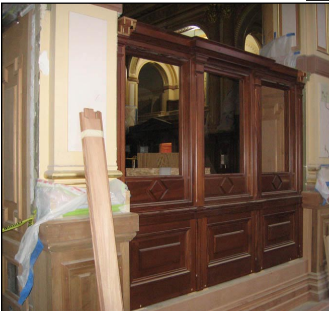
New side walls from side corridor.
