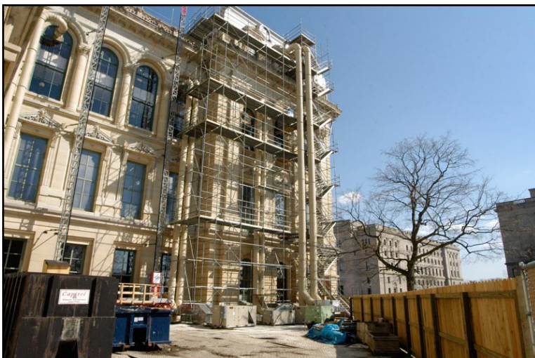
View of construction from the outside.
