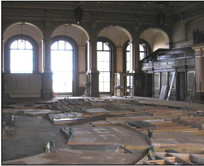
Overall view of chamber under construction.
