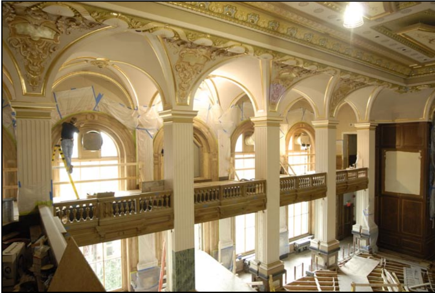
Cleaners and filters were installed as the HVAC system was modernized.
