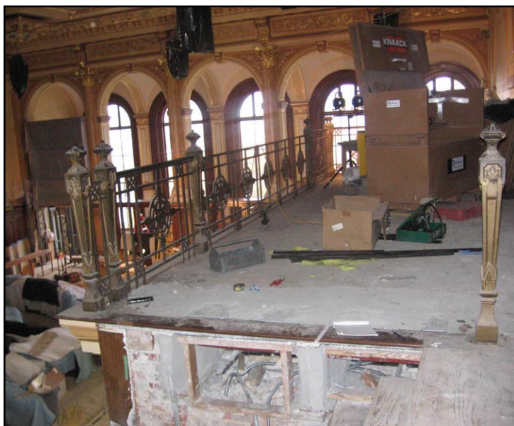
South Gallery railing being removed.
