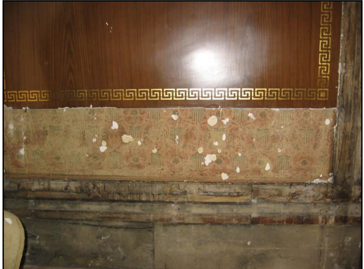
Stencils discovered on north wall of chamber.
