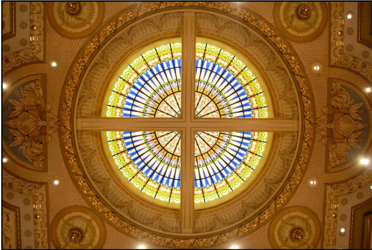
The newly installed laylight in the House ceiling.
